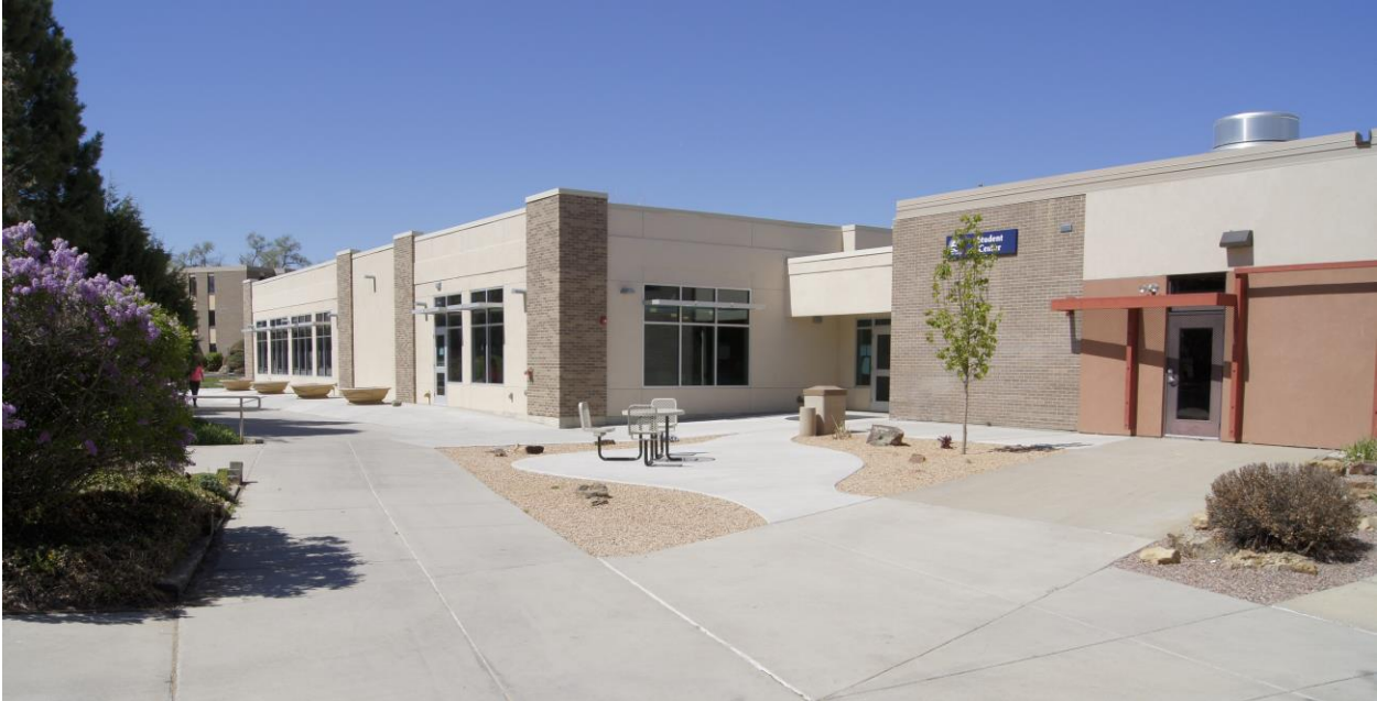
Student Center 1966 -remodeled 2013: Interior remodels and additions have occurred. Exterior might need CHS review.
