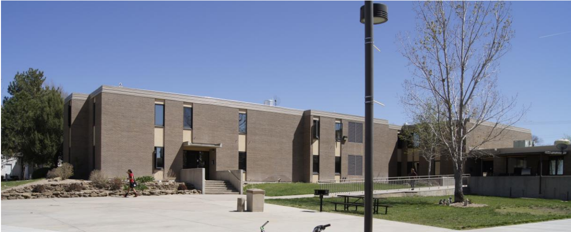
Wunsch Hall 1966 -remodeled 2001-2015: Interior remodels only have occurred. Exterior might need CHS review.
